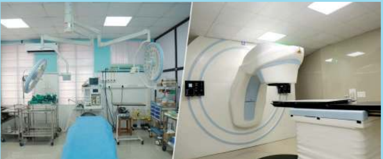
Burns Treatment Unit
